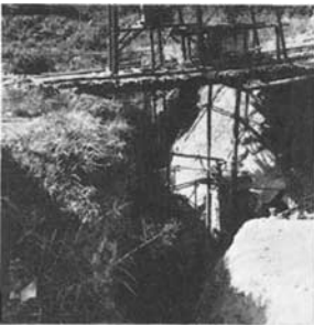
FIG. 5. At Tawmaw wide and deep vertical shafts are sunk down to the jadeite dykes. Here a primitive lift is operated from a simple bridge consisting of jungle wood beams and bamboo rods.
