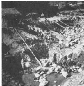
FIG. 7. Details of the river mining at Hpakant . Small claim in the foreground. Machine pump hoists ground water through metal hose back into the river.
