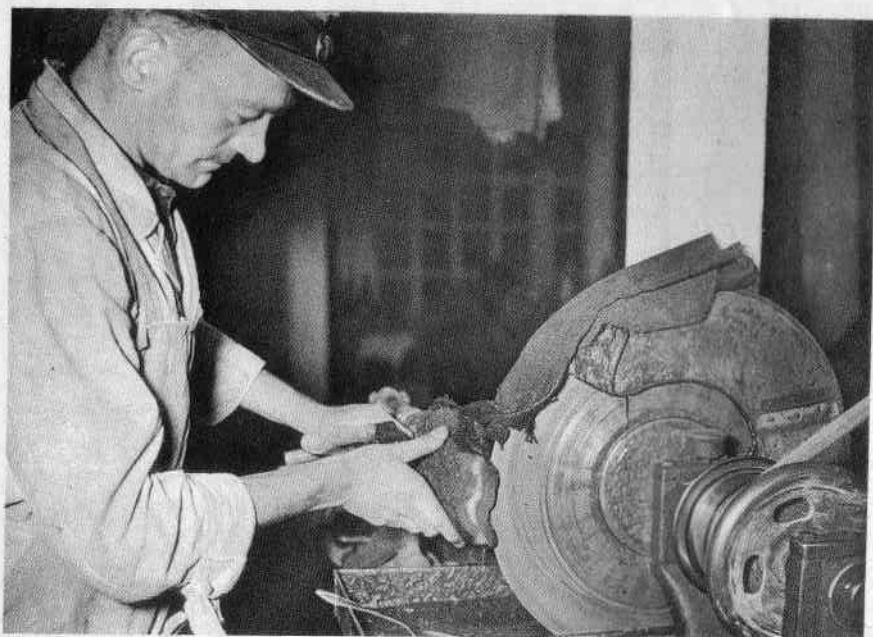
The only modern equipment in the shop is this electrically driven slabbing saw.
