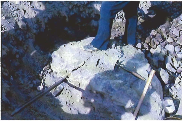
Figure 4. Tools used to break the fractured basalt into small chunks.
