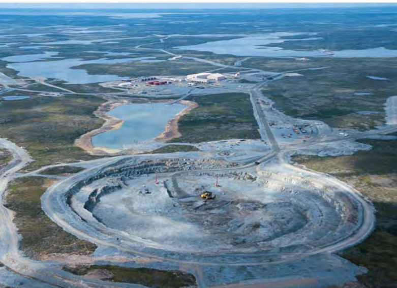
Figure 3. This aerial photograph of the Ekati diamond mine, looking south (with the camp and processing facilities in the distance), was taken in August 1998. The Panda pit (foreground) measures about 900 m in diameter; the kimberlite is the much smaller dark region in the center and lower right of the pit floor. (The area of the pit is larger than the pipe because of the requirements of open-pit mining.) Eventually, the bottom of the pit will be about 100 m wide and 300 m below the present surface, at which time underground mining will commence. Just beyond the Panda pit is Koala Lake, which marks the location of another kimberlite that is scheduled to begin mining in 2002. Photo © Jiri Hermann/BHP Diamonds Inc.
