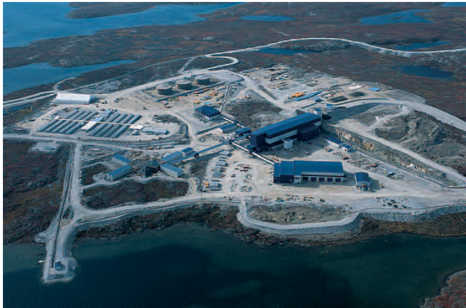
Figure 13. This aerial view of the Diavik mine was taken in September 2002. The large (11 story) building in the center is the processing facility, where diamonds will be separated from the kimberlite host rock. The building to the lower right serves as the maintenance and administration center. In the lower left is the permanent accommodations facility, and above it (with the smoke stacks) is the power plant. Photo by Jiri Hermann; courtesy of Diavik Diamond Mines Inc.
