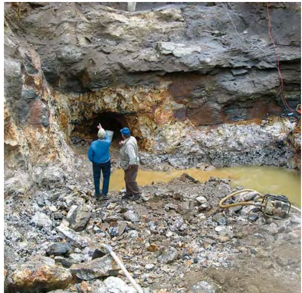
Figure 8. The entrance to a large pocket (no. 7) containing mostly green tourmaline is marked by the small tunnel just in front of the men in the pit. Note the location of this pocket within a pronounced bulge in the thickness of the predominantly light-colored pegmatite. Photo by Alexander Falster.
