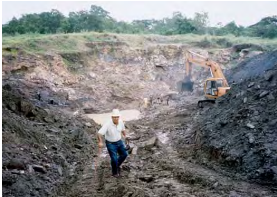
Figure 4. Canary Mining Ltd. used a large excavator to explore primary deposits from December 2003 to August 2004. The main pegmatite is being mined down-dip from the area that produced large amounts of tourmaline in the mid-1990s; Asok Napa (in the foreground) was the mine's general manager during that time. Photo by Tommy Wu.
