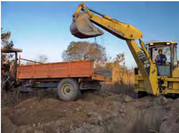
Figure 13. Mozambique Gems is digging this test pit to help determine the extent of the tourmaline-bearing layer on their concession. The material from the gem-bearing layer of the pit will be washed, screened, and hand-picked for tourmaline. Photo by B. M. Laurs.
