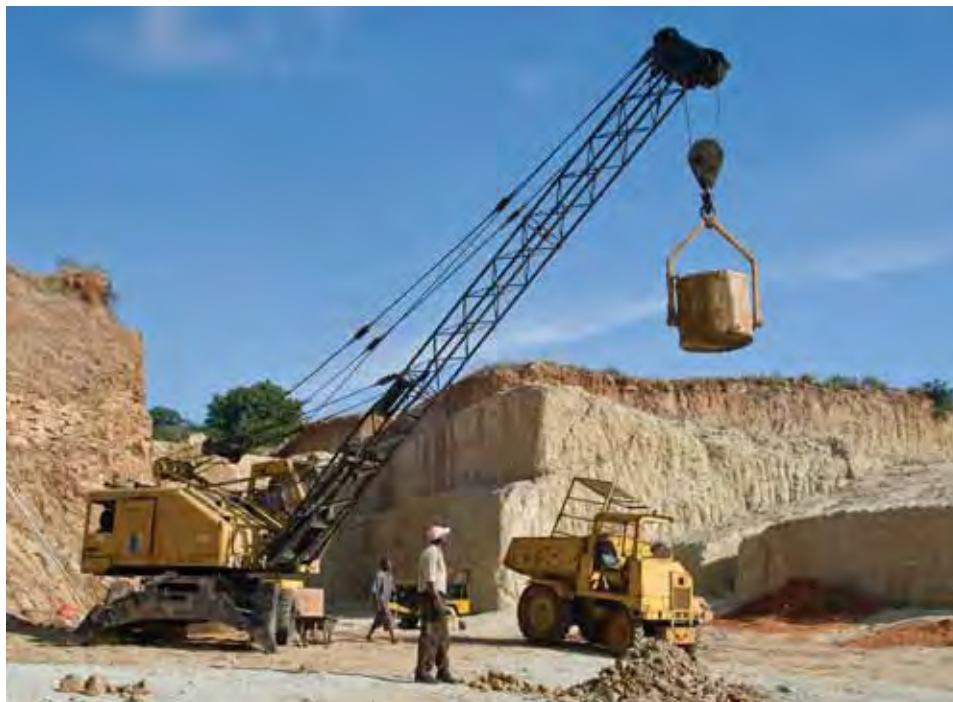
Figure 16. Cranes are used to remove the excavated material from the shafts, as shown here at the Kimbo pit. A cage that is used for hoisting the miners is visible in the dump truck. Photo by B. M. Laurs.
