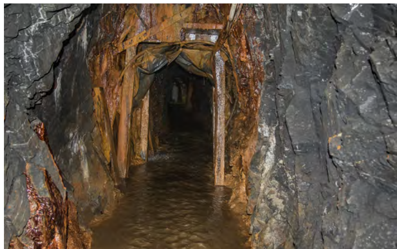
Figure 10. Flooding is a constant struggle in many of Colombia's mining tunnels. Shafts can rapidly fill with water, and the tunnels often have streams of water running through them. Photo by Andrew Lucas.
