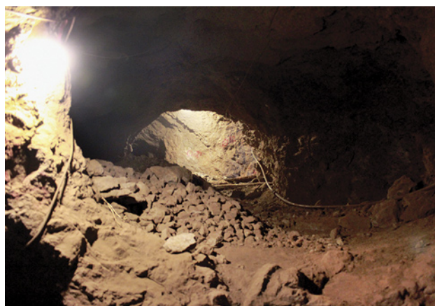
Figure 9. A raise in the form of an inclined path up to the higher levels. Photo by B. Shirdam.
