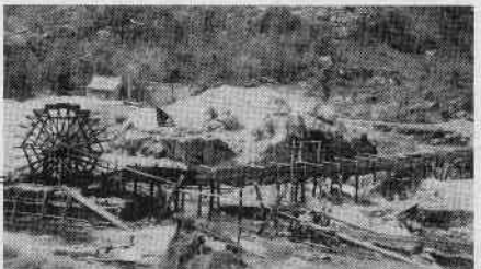
● Undershot wheel, turned by power from flume water, is used to keep pit dry between two dams. Pipes in foreground carry away seepage.
