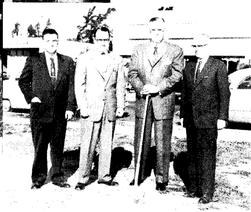
Turning the ground for the new building. Reading from left to right are Allan D. Gill, Richard T. Liddicoat, Jr., James G. Donovan and Fred J. Cannon.
