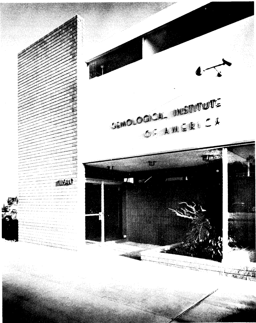
Front entrance from San Vicente Boulevard, facing north.
