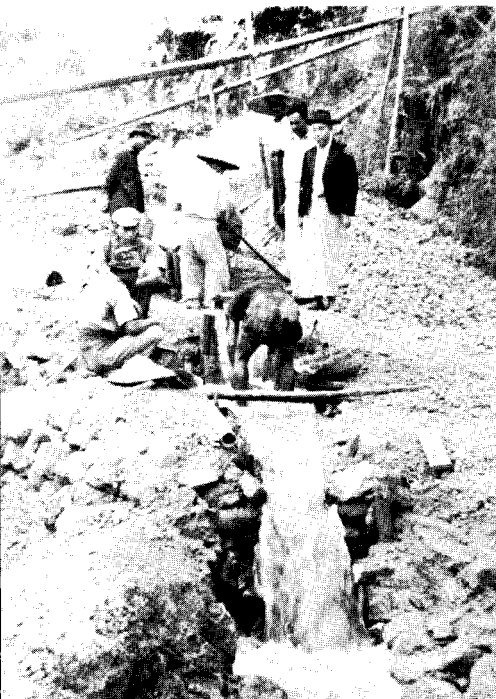
• Recovering gravels falling over the series of falls.
