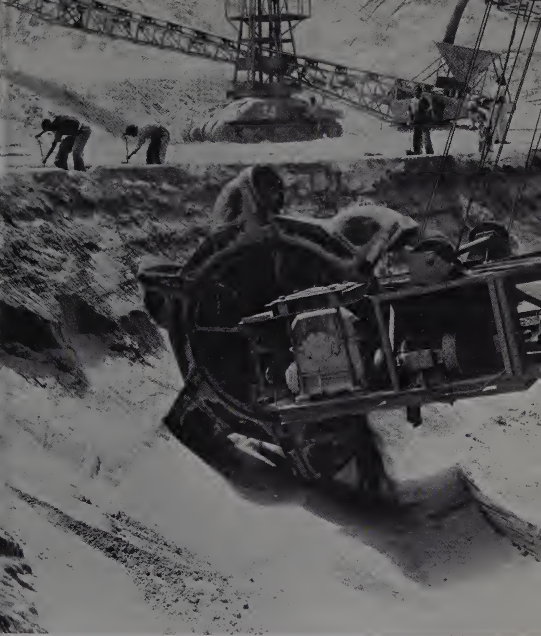
Removing the overburden covering diamondiferous gravels on coast of South West Africa. Rotary bucket excavators remove 660 tons of sand per hour, which is conveyed to disposal areas. After clearing the sand, mining of the diamondiferous gravels can begin. See page 42.
