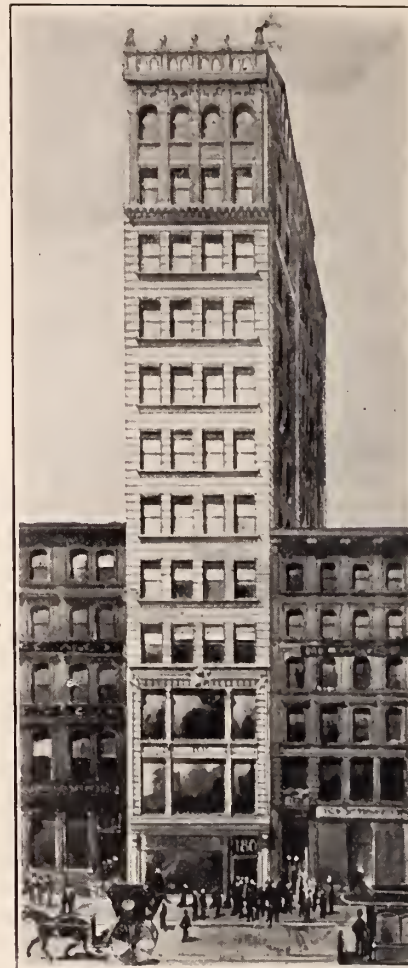
BUILDING BEING ERECTED FOR JEWELERS AT 180 BROADWAY, NEW YORK.
