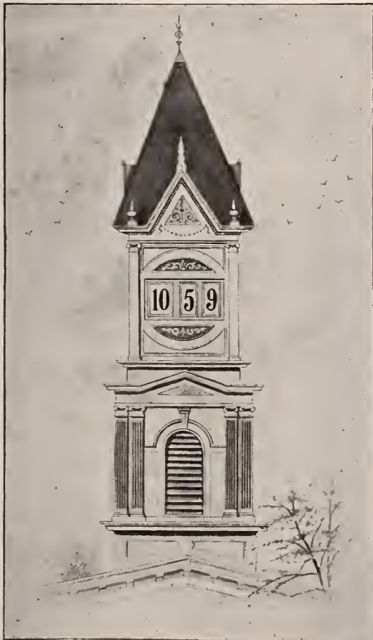
THE THRASHER TOWER CLOCK TO BE OPERATED BY A MASTER CLOCK LOCATED WHERE IT WILL BE FREE FROM VIBRATION.
