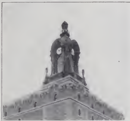
CLOCK ON LONG ISLAND STORAGE WAREHOUSE.
