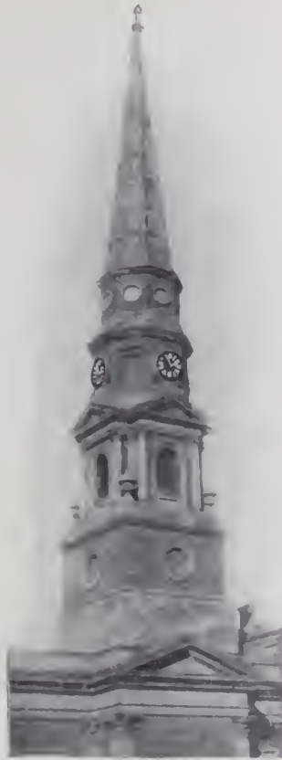
BRICK CHURCH CLOCK.
