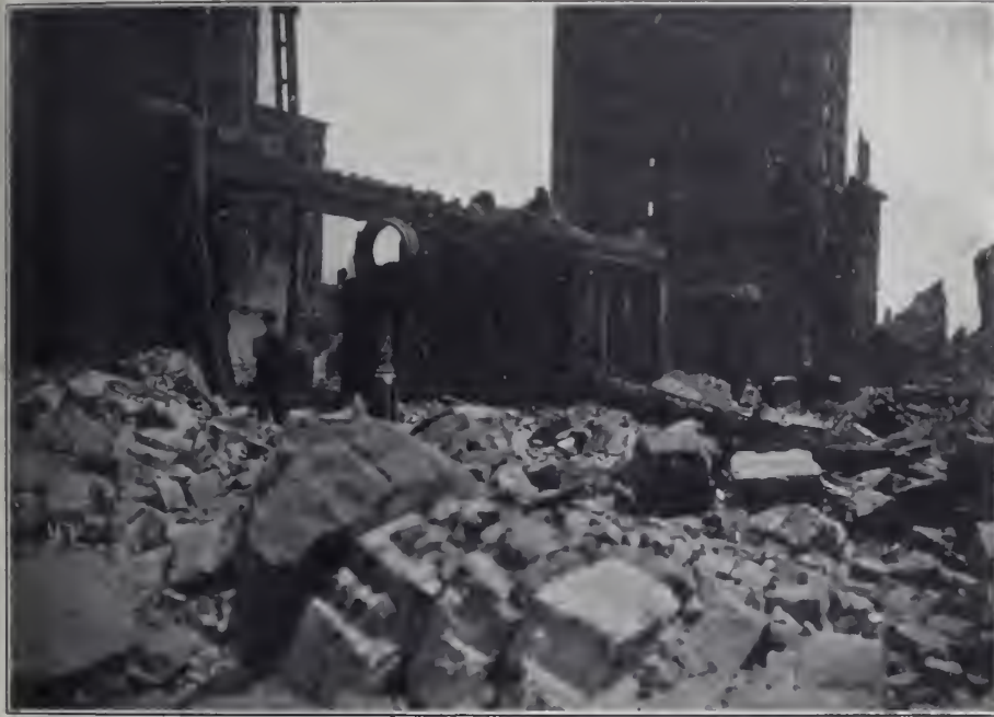
LEVINSON BUILDING, SHOWING RUINS OF STORES OF W. K. VANDERSLICE CO. AND CALIFORNIA JEWELRY CO.
