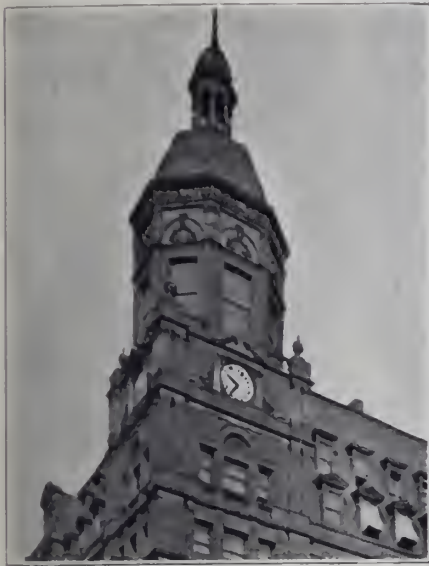
CLOCK ON THE GARFIELD BUILDING.
