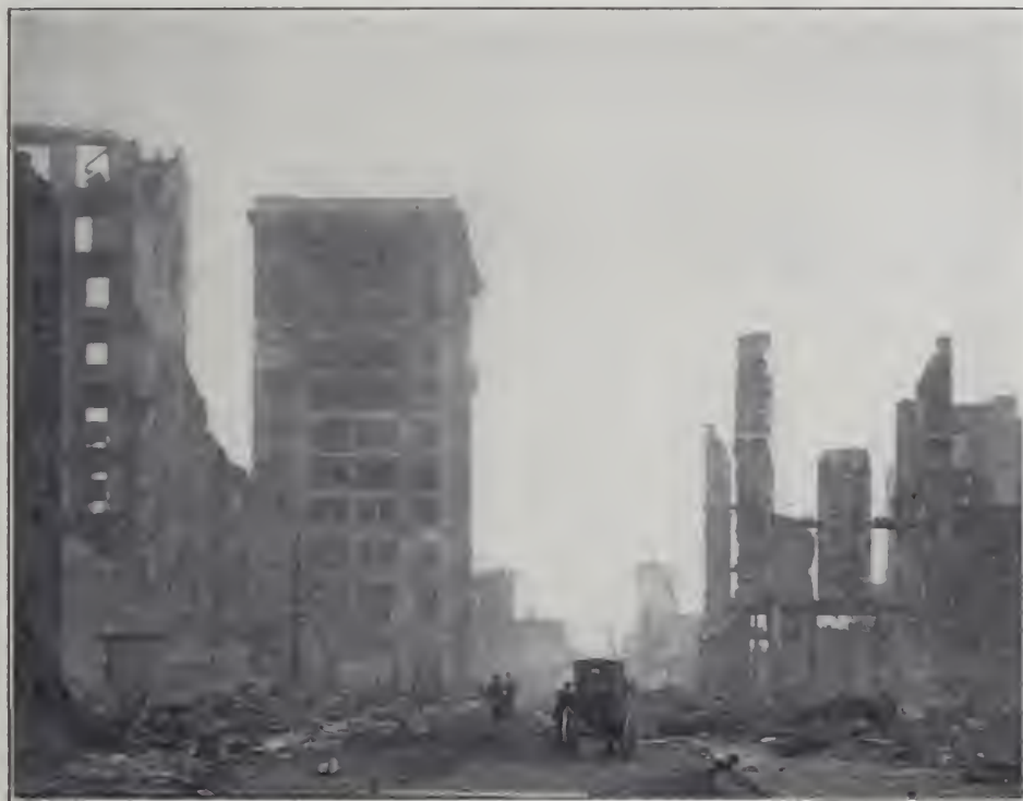
HOW THE SHREVE BUILDING NOW LOOKS, WITH ITS WALLS AND FLOORS STILL IN GOOD STATE OF PRESERVATION.
