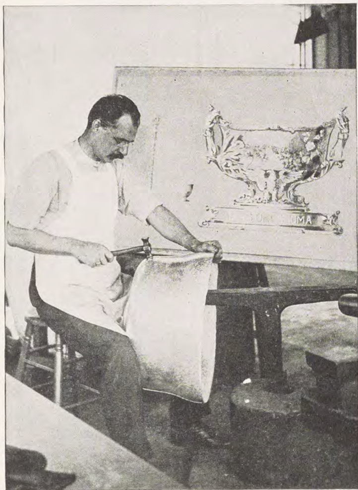
FIG. 137. SILVER PUNCH BOWL FOR U. S. BATTLESHIP "OKLAHOMA" IN PROCESS OF BEING RAISED
