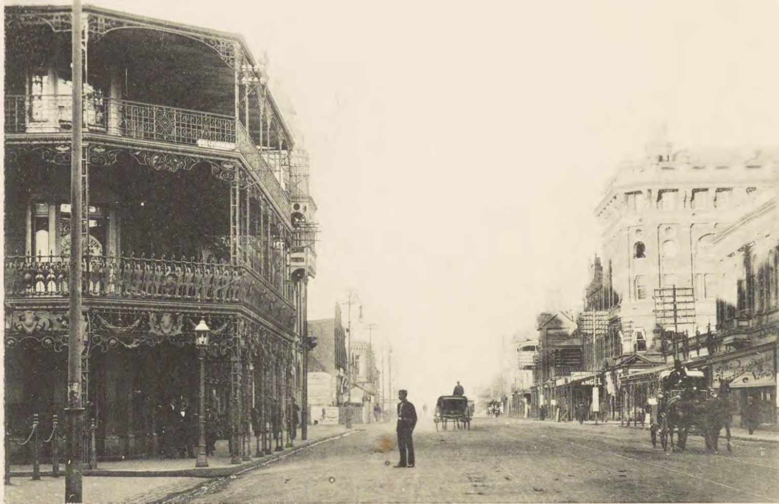
26. Commissioner Street, looking West.
