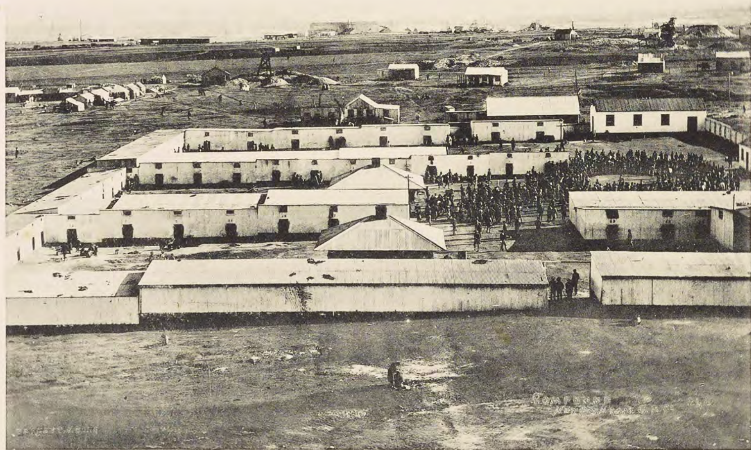
56. The Compound. The New Primrose Mine.
