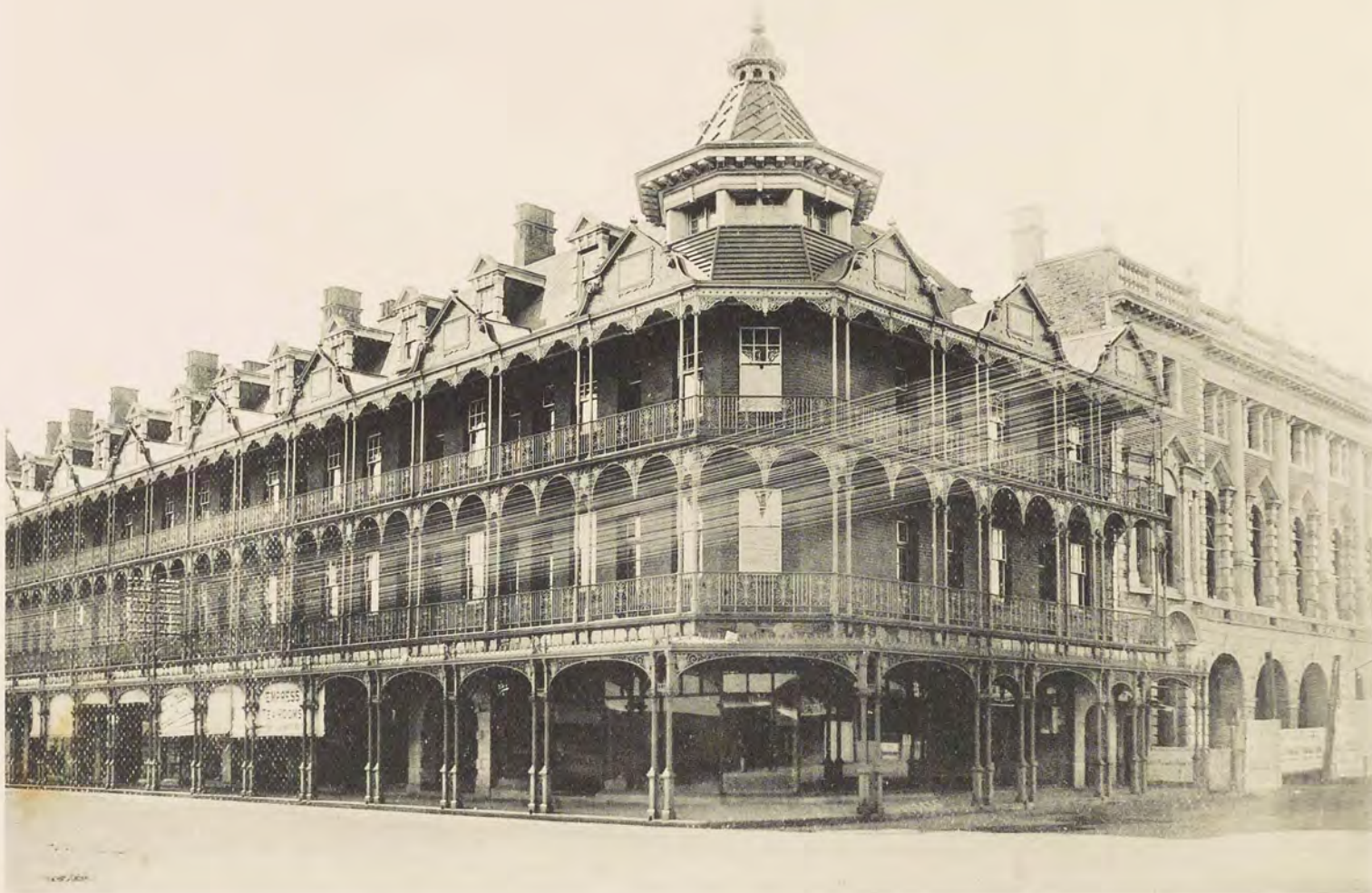
22. Pollock Buildings, Eloff Street, showing portion of New Library.
