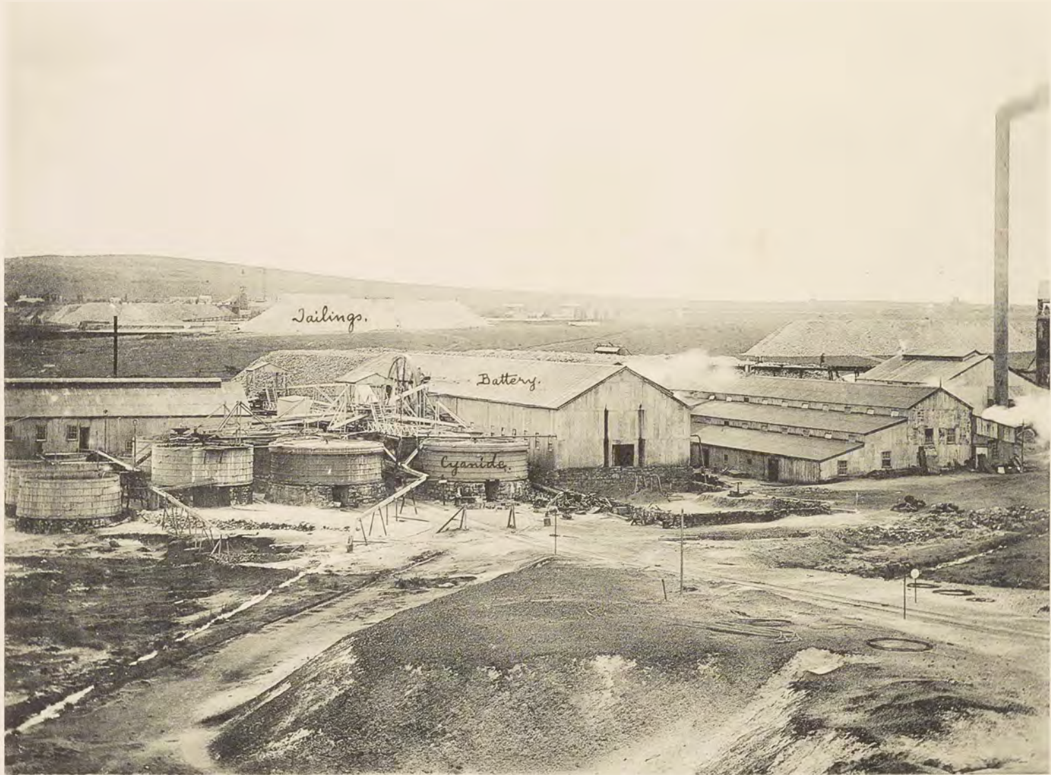
44. Battery and Surface Works, the Jumpers Mine.
