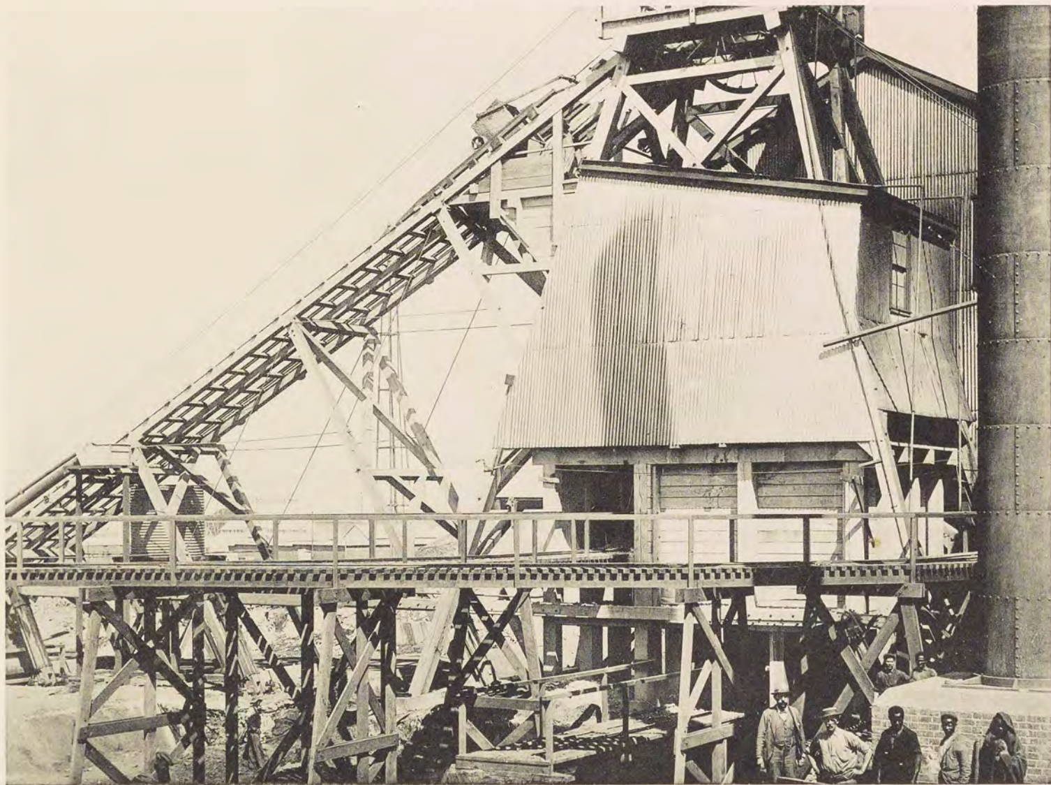
43. New Headgear, Simmer and Jack Mine.
