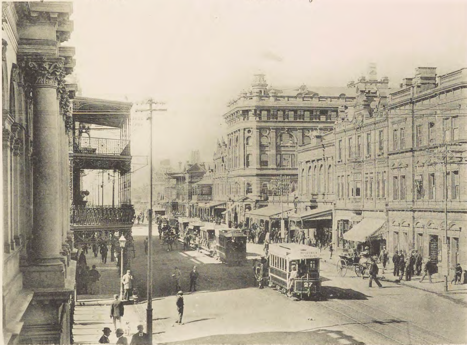
25. Commissioner Street, looking West.
