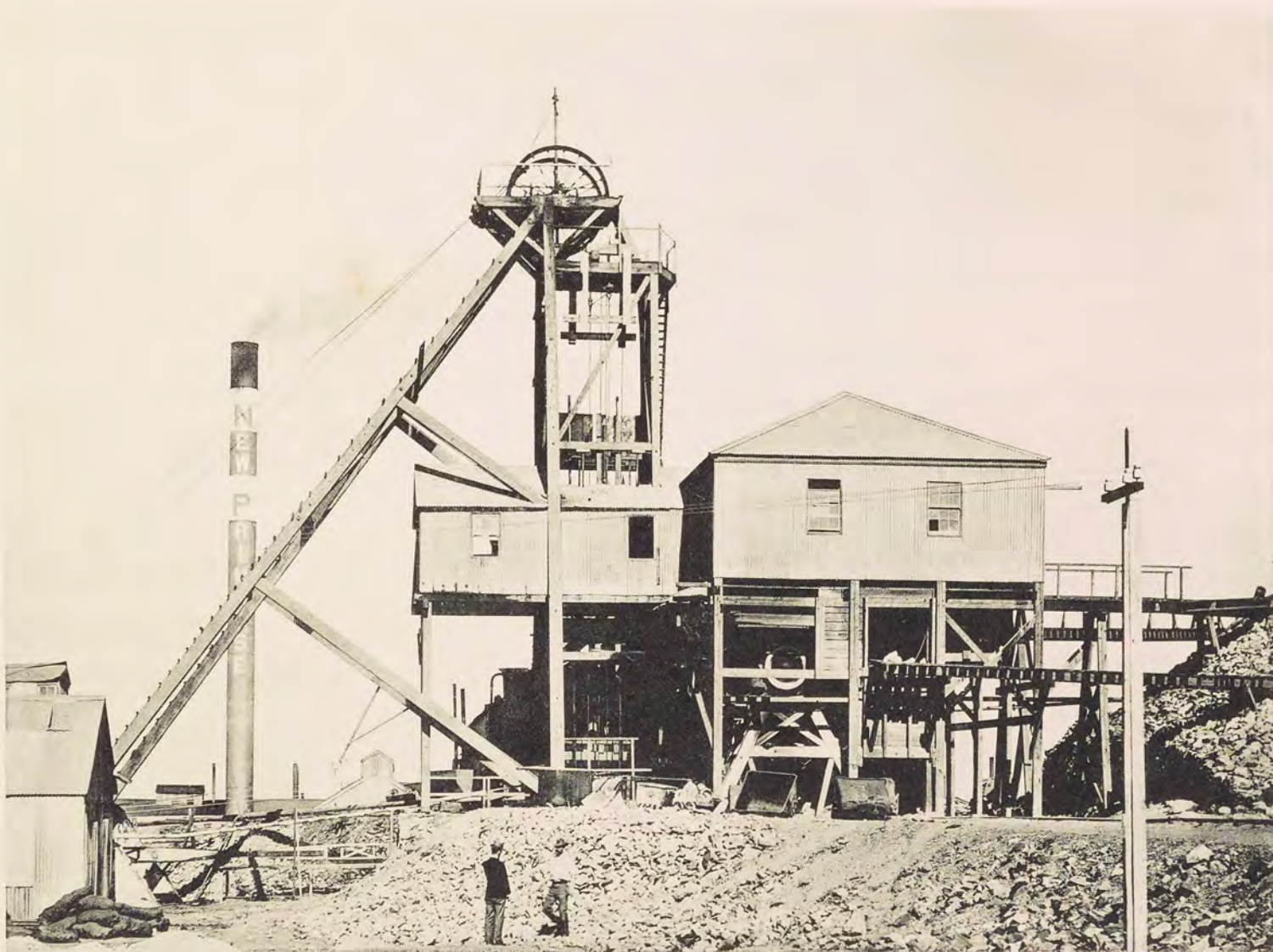
45. Headgear and Surface Works, the New Primrose Mine.
