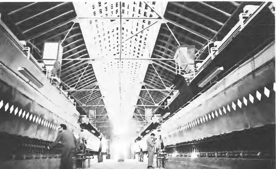
Fig. 2.5 (c) One of the furnace rooms at Monthey.
