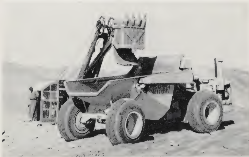
Fig. 11—Ten-ton rear dump truck and 38 cu. ft. excavator
