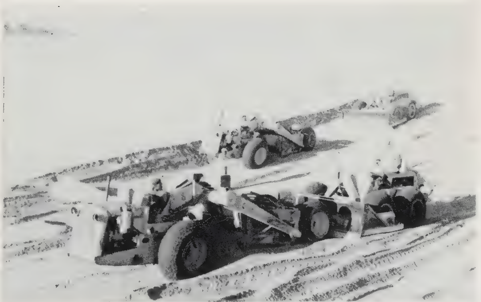
Fig. 7—Pneumatic tyred scraper and bulldozer in action
