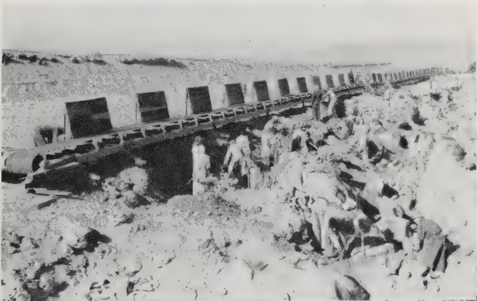
Fig. 2—Bedrock cleaning
