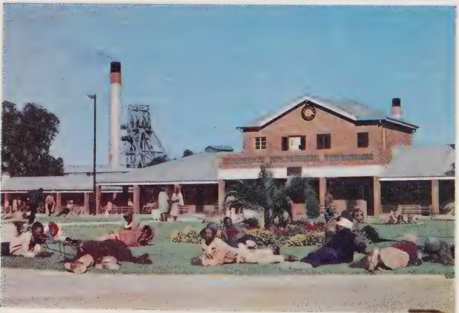
Fig. 1—The Administration Block at Dutoitspan Hostel with the mine headgear in the background
