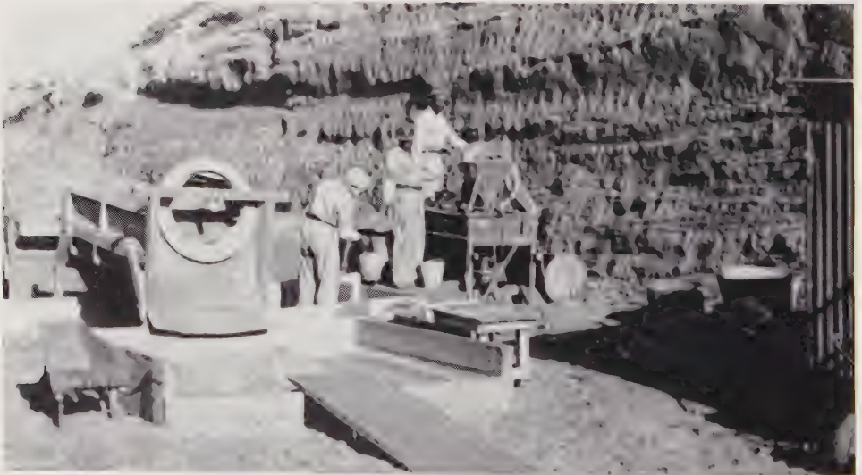
Fig. 4—Classifying trommel and jig
