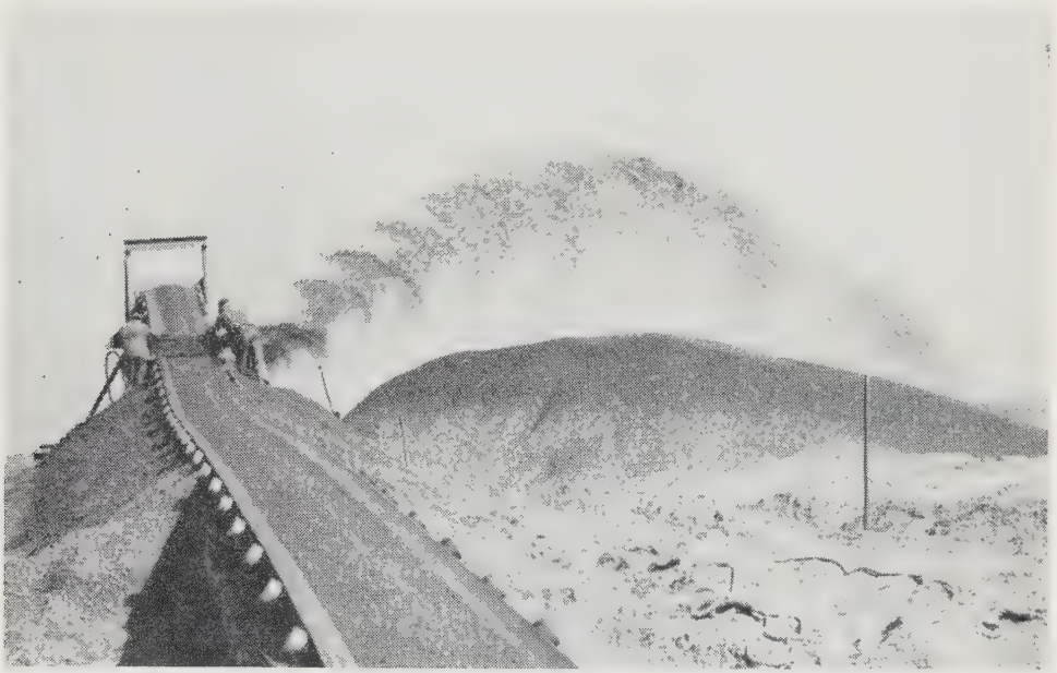
Fig. 8—Tailings disposal by flinger
