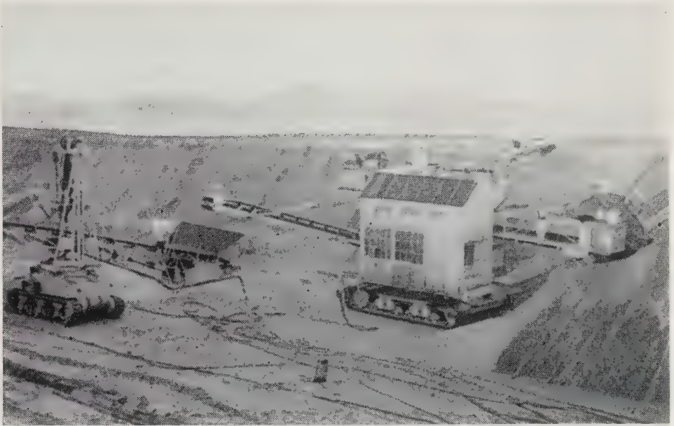
Fig. 6—Bucket-wheel excavator with stacker
