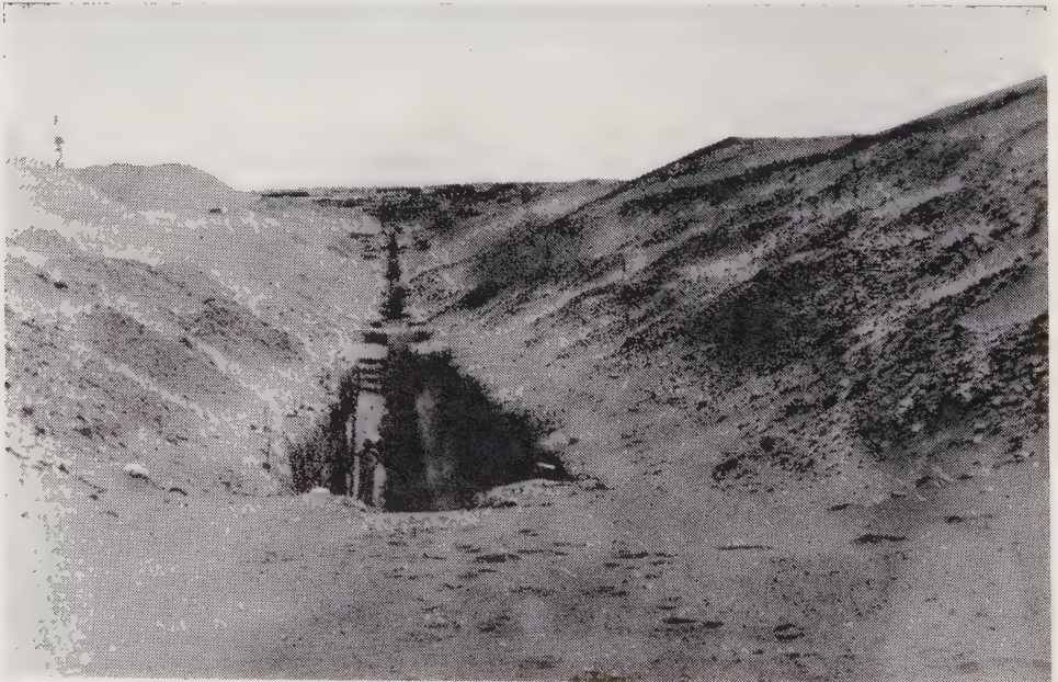
Fig. 1—Sampling trench and sand overburden
