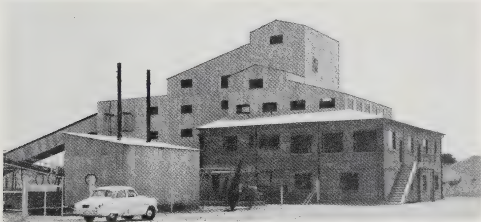
Fig. 12—Exterior view of recovery plant
