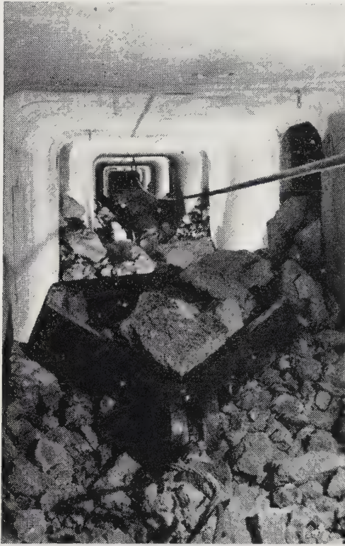
Fig. 16—Scraping in a drift
