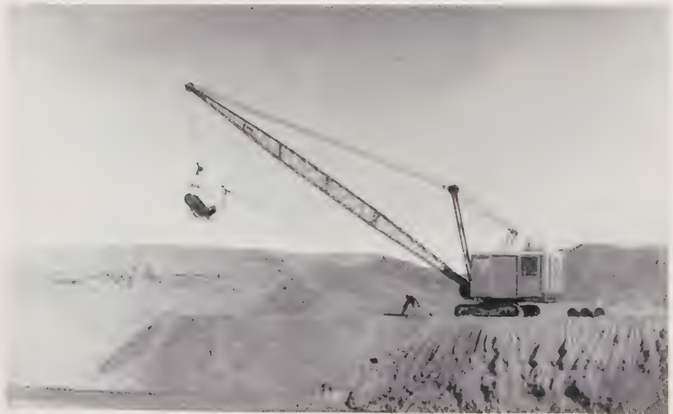
Fig. 9—Dragline excavator in action
