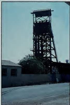
3 Underground mines are usually off limits to collectors, but many miners manage to salvage specimens (at some risk to their jobs). Head frame at Tsumeb, Namibia.
