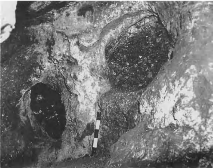
Fig. 8: Mine 2 at Aghios Sostis on the Cycladic island of Siphnos (Greece). The two galleries of the Early Cycladic period were exposed by blasting during the 19th and early 20th century mining for iron ore. Their oval section is typical for the use of firesetting and heavy stone mauls.
