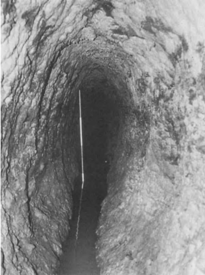
Fig. 16: Cross-cut gallery G8 driven to drain Les Fouilloux gold mine.
