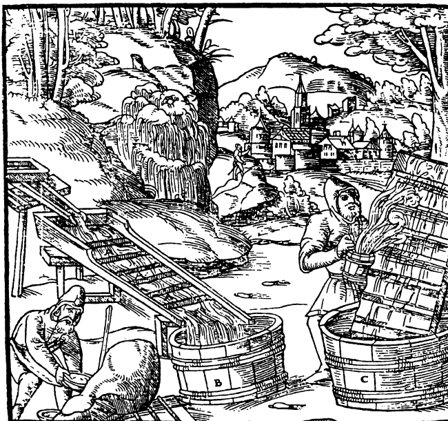
Fig. 1: The technique of extracting fluvial gold in the sixteenth century. The gold-bearing sand is shovelled onto the sluice box (A), where the gold "tinsel" collects in the transversal grooves. The concentrate is rinsed in a tub (C), and then washed out presumably using pans. After Georgius Agricola, De re metallica (1556).
