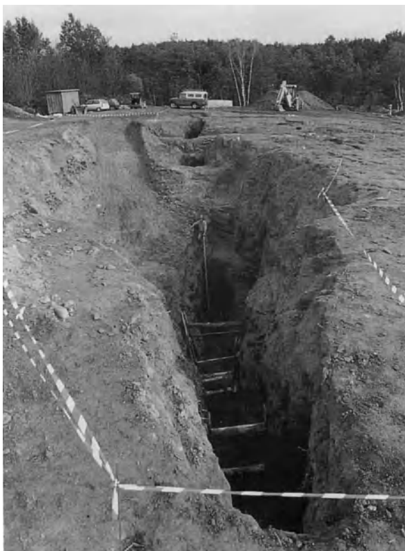
Fig. 9: Stope F9 at Cros Gallet-Nord worked by simple underhand stopes.
