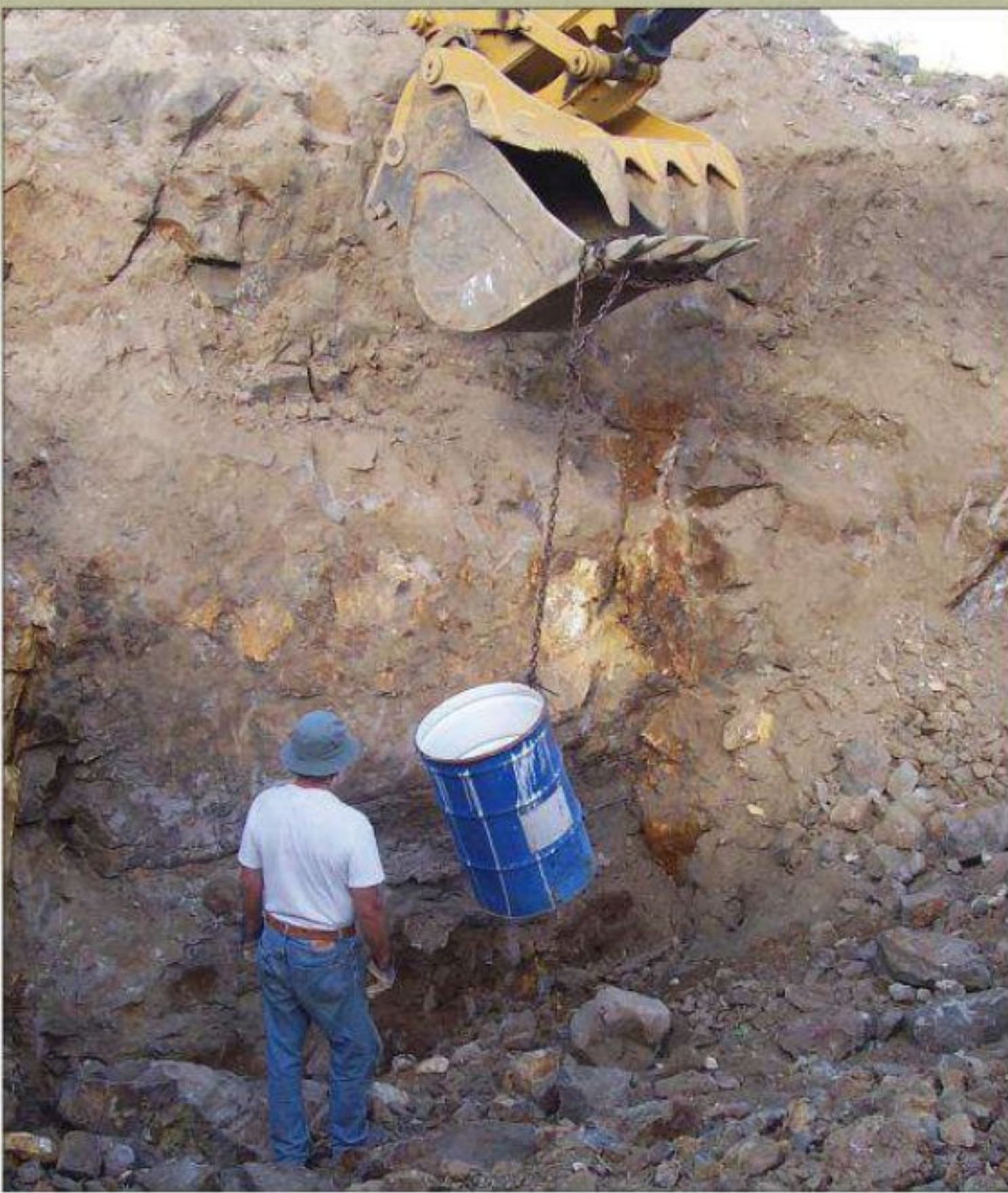
Gene fashioned a muck bucket out of a 55-gallon steel drum and used it to help dig out backfill from the cave he had discovered in 2007.
