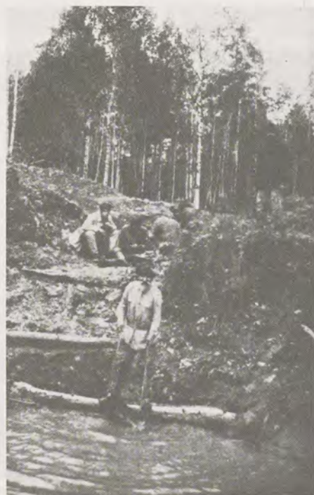
Fig. 14-60 Top: prospect pits being opened in the forest near the Stretensky emerald mine, Urals. Bottom left: a long trench dug to expose bedrock in order to aid in mapping the geology of the emerald formations. Bottom right: washing samples of emerald-bearing rock. Photos by A. E. Fersman, "Smaragdgruben im Uralgebirge," Abhandlungen zur praktischer Geologischer und Bergwirtschaftslehre 18, part 1 (Halle, 1929).
