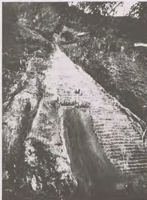
Fig. 14-26 Views taken in the Chivor emerald mine about 1920, showing clearing of overburden (top photos) and development of the "step" or "benching" method to systematically excavate the emerald-bearing ground. From L. J. Canova, Chivor-Somonoco Emerald Mines of Colombia (New York, 1921).
