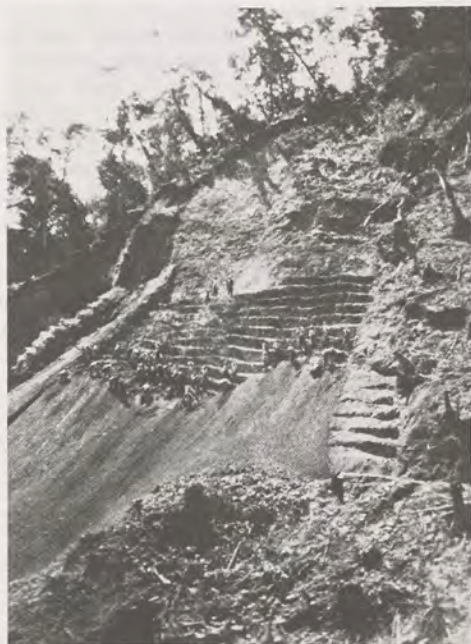
Fig. 14-26 Views taken in the Chivor emerald mine about 1920, showing clearing of overburden (top photos) and development of the "step" or "benching" method to systematically excavate the emerald-bearing ground. From L. J. Canova, Chivor-Somonoco Emerald Mines of Colombia (New York, 1921).
