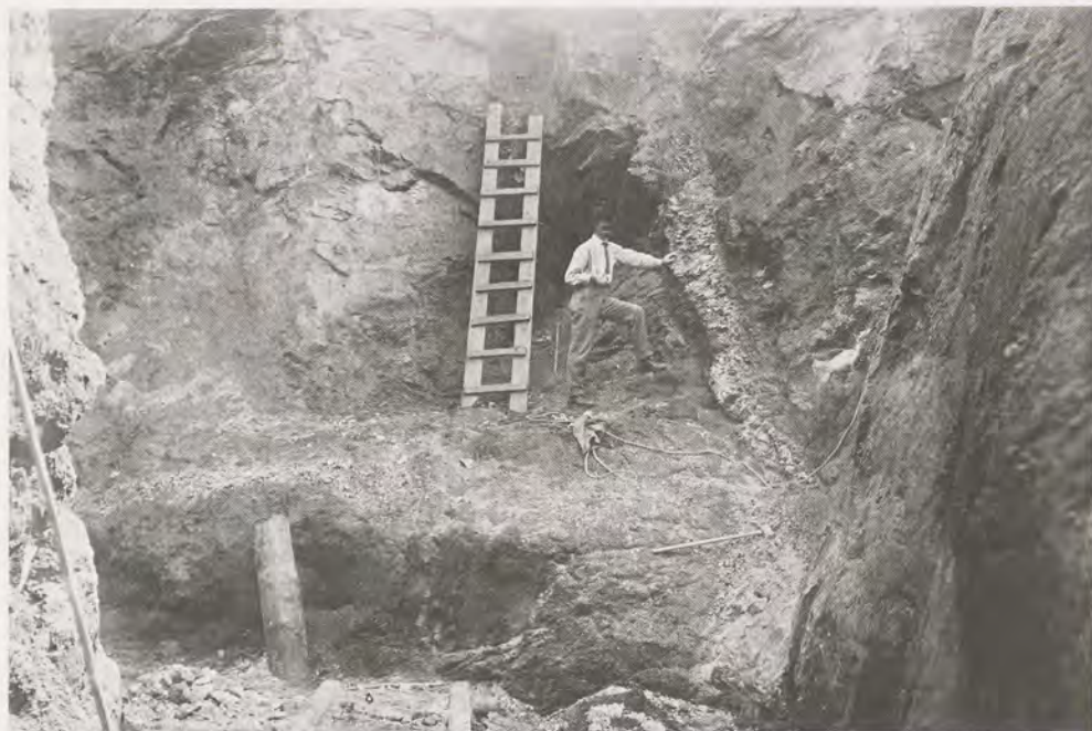
Fig. 14-72 Turner emerald mine near Shelby, North Carolina, 1912. The emerald-bearing pegmatite dike is to the right and appears as a crumbling feldspar streak passing almost vertically through the decomposed gneissic country rock. Courtesy U. S. Geological Survey.
