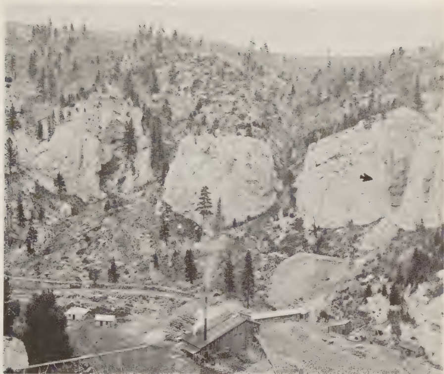
FIGURE 120. The American Sapphire Mine in Yogo Gulch, Montana in 1912; view looking northeast across the gulch. The steep cliffs are limestone and this is the rock in which the sapphire-bearing dike is intruded. At the extreme right, as marked by the arrow, the narrow defile created by removal of the dike rock is still to be seen. Courtesy U. S. Geological Survey.
