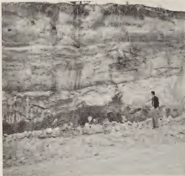
FIGURE 76. Residual bauxite being mined as an ore of aluminum near the Sweet-water Branch, Andersonville, Georgia. The man is standing on a bed of bauxite four feet in thickness which has been covered by an overburden of sediments measuring about 20 feet in depth. Courtesy U. S. Geological Survey.
