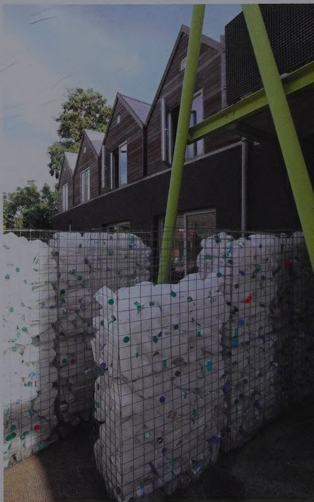
Milk Container Wall , Julia Manheim/Ken Taylor, 2006. Plastic milk containers, steel gabions. Photo: Anthony Coleman
