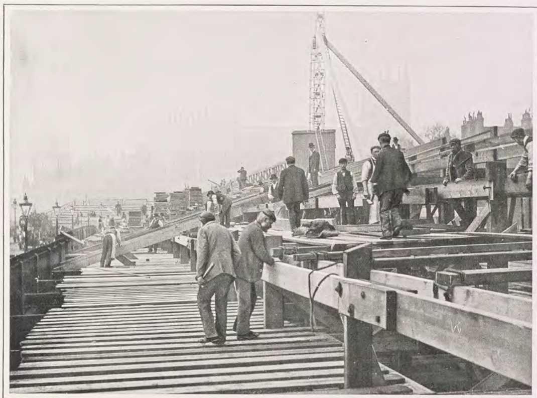
ERECTING ONE OF THE GRAND STANDS AT WESTMINSTER.
