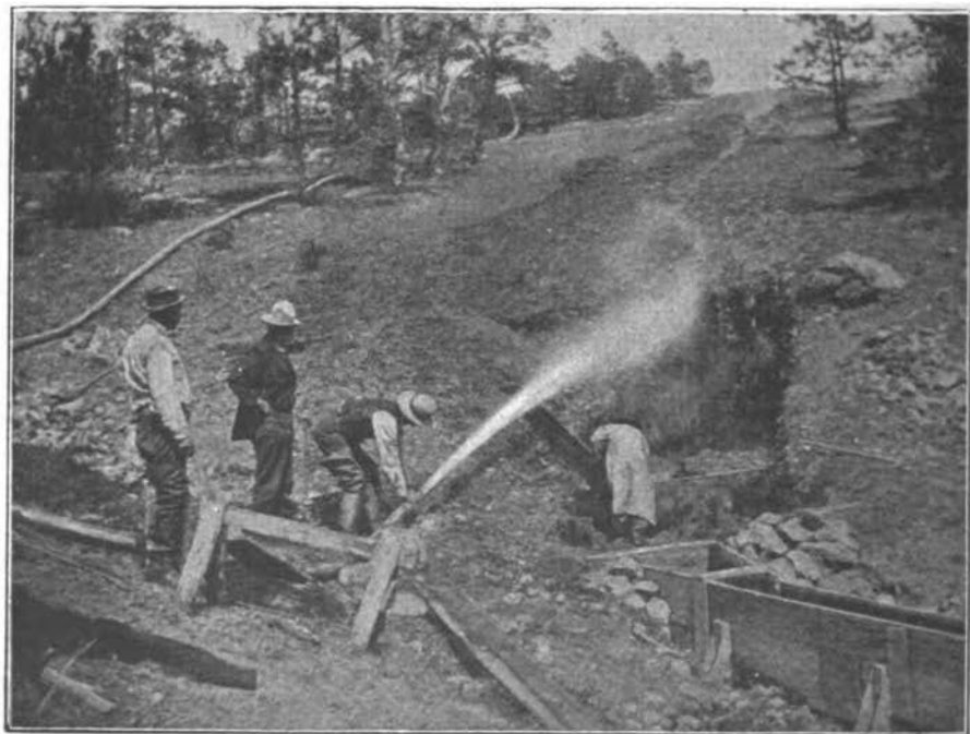
MONTANA SAPPHIRE MINING—A "NEW CUT."
