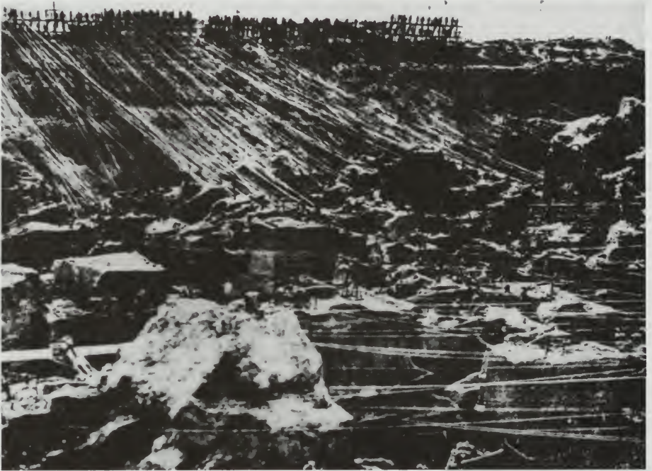
The Kimberley Mine in the 1880s. The ropes crisscrossing from the rim on the kimberlite pipe run to thousands of individual claims below. Courtesy of De Beers.
