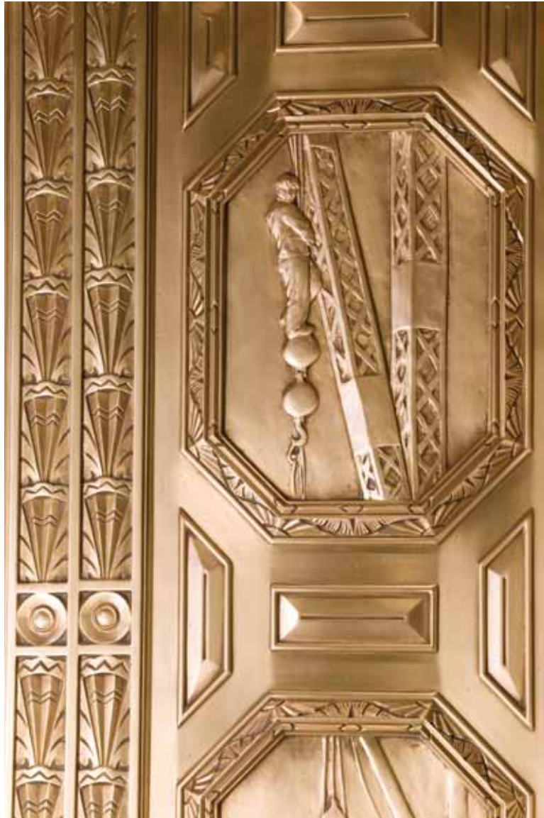
Figure B1. Detail photograph of bronze paneled lobby elevator door, Fuller Building, New York, NY. An advertisement for the General Bronze Corporation in the March 1930 issue of Metalcraft states that the casting of these doors was executed at the John Polachek and Tiffany Studios foundry in Corona, Long Island. Photograph Courtesy of the current owners of the building: Vornado Office Management, LLC.
