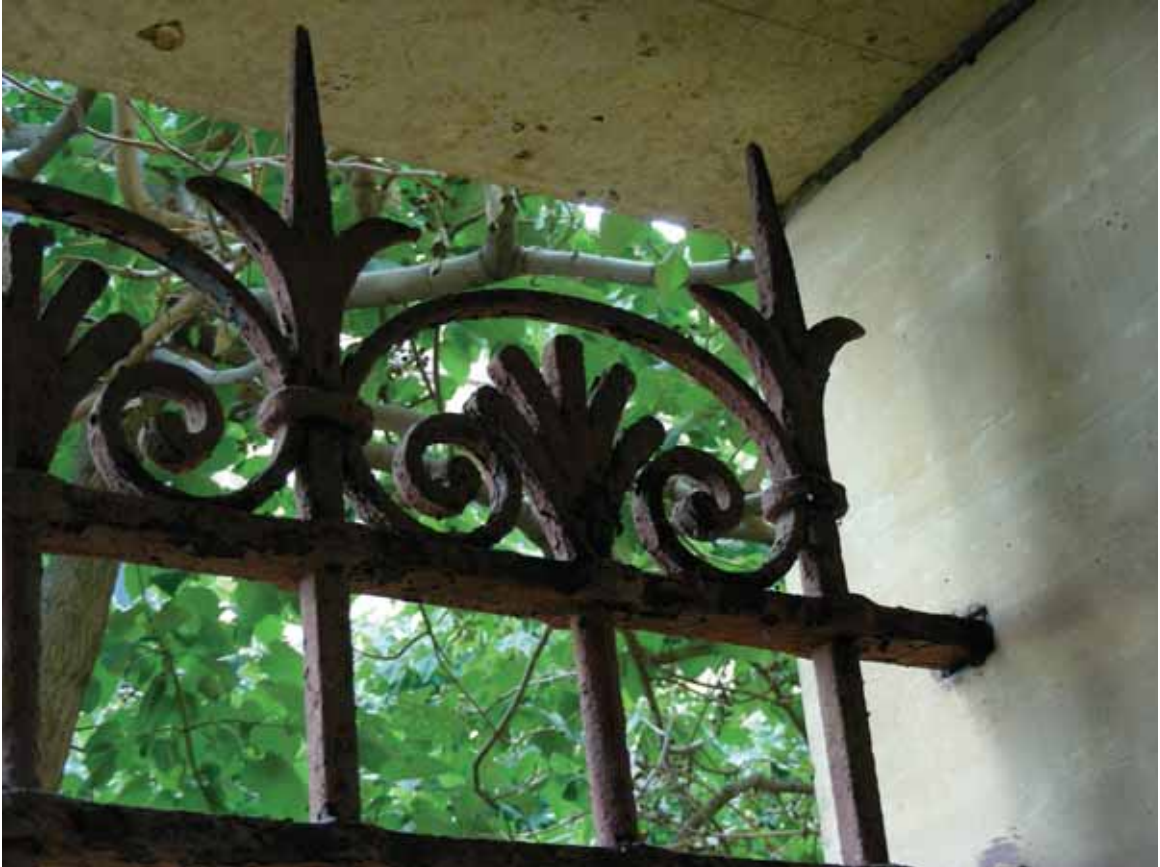
Figure C2. Iron grilles before conservation treatment, with the most recent paint layer, a red brown. Photograph courtesy of Melissa S. Meighan, PMA.
