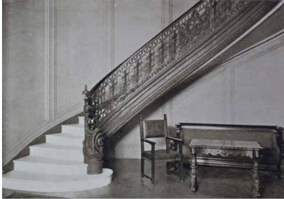
Figure 4.1. “Bronze Stair Railing Executed by Tiffany Studios”. Photograph from Character and Individuality in Decorations and Furnishings , published by Tiffany Studios 1913. Courtesy of the Louis Comfort Tiffany Collection at the Charles Hosmer Morse Museum of American Art Archives.
