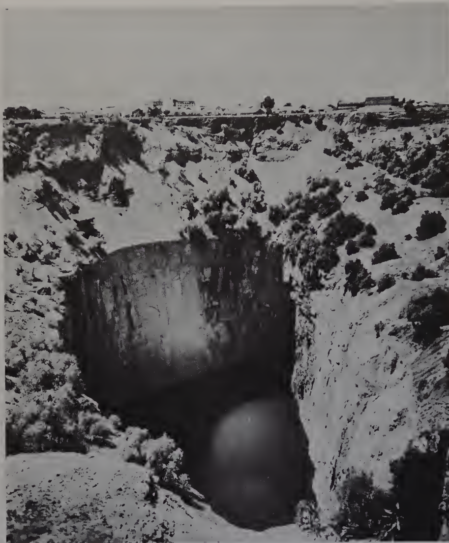
The Kimberley Mine or "Big Hole" in South Africa had reached 1,000 feet when this picture was taken in 1876. Before it was shut down in 1960 and water allowed to fill the bottom, it was 3,520 feet deep and 1,520 feet across. It is the largest man-made crater in the world.
