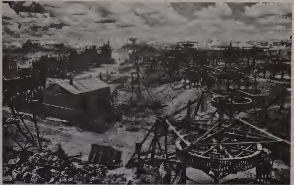
Topside at Kimberley the ore was sifted by horse-power.
