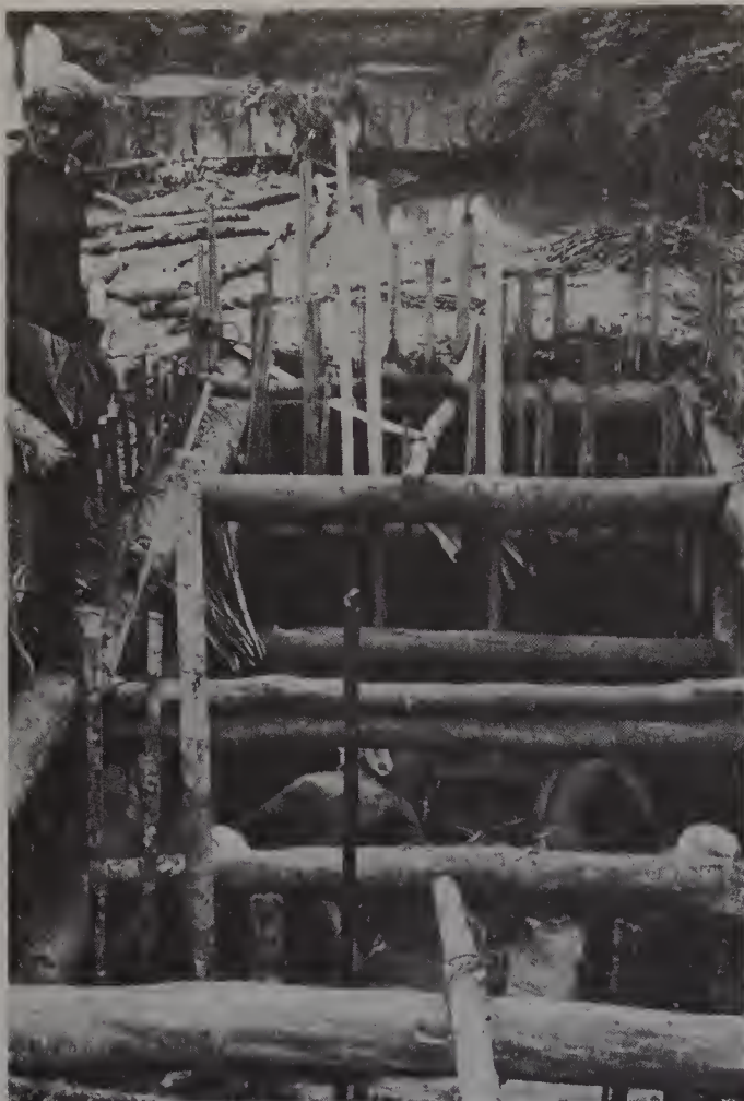
(Left) In some areas of Sri Lanka (Ceylon) there are gravels about 30 feet (9 meters) below the surface containing ruby, sapphire, garnet, topaz, zircon, tourmaline, spinel and many other gems except diamond. They are mined by making shored pits and winching up gravel baskets filled by men below. (Right) The sandy gravel is washed and swilled in these baskets to remove the sand and lighter elements so that the precious stones, which are generally heavier, remain and can be picked out.
