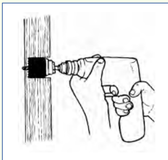
FIGURE 54 —Cut the hole for the doorknob using a hole saw attachment on an electric drill.
