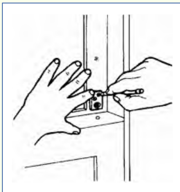
FIGURE 85 —Drill the holes for the bolt and the strike screws.
