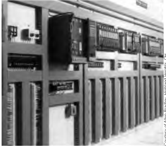
Figure 20-3. Placement of PLC components.
