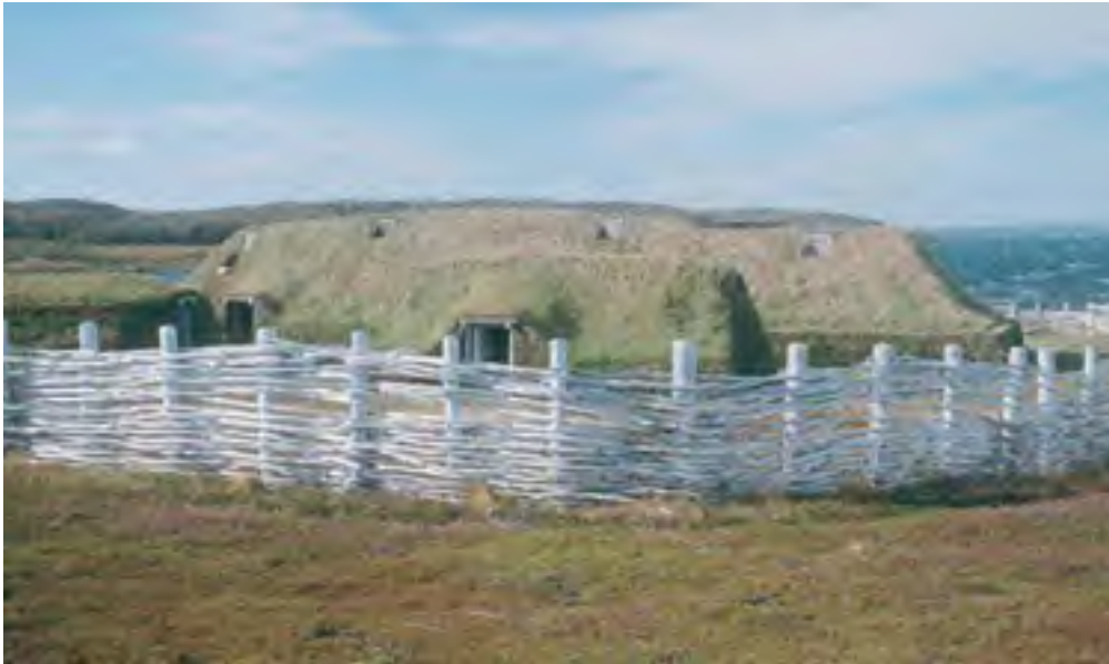
Viking Longhouse. A simple turf bunker was built by the Vikings on the coast of Canada. Low-lying for protection against wind and snow, it was built as a permanent settlement and trading post with the Eskimos. Viking trade goods appear far to the north in Baffin Island.
