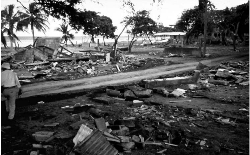
Figure 5.16. El Tránsito, Nicaragua after the tsunami of September 2, 1992. While the second wave, which was 9 m high at this site, destroyed most of the houses, only 16 out of 1,000 people died because most fled following the arrival of the first wave, which was much smaller. Photo credit: Harry Yeh, University of Washington. Source: NOAA National Geophysical Data Center.
