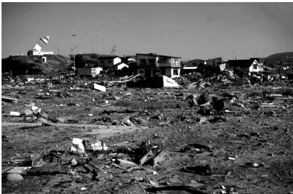
Figure 5.19. Damage at Aonae, Okushiri Island, due to the Hokkaido Nansei–Oki tsunami of July 12, 1993. The earthquake, and not the tsunami, damaged the leaning lighthouse. Concrete foundations in the foreground have been wiped clear of shops, houses, and kiosks. Note the gravel and boulder dump deposit, and the similarity of the unit to that deposited by the Flores tsunami in Figure 3.6. Photo credit: Dennis J. Sigrist, International Tsunami Information Center at Honolulu, Hawaii. Source: National Geophysical Data Center.
