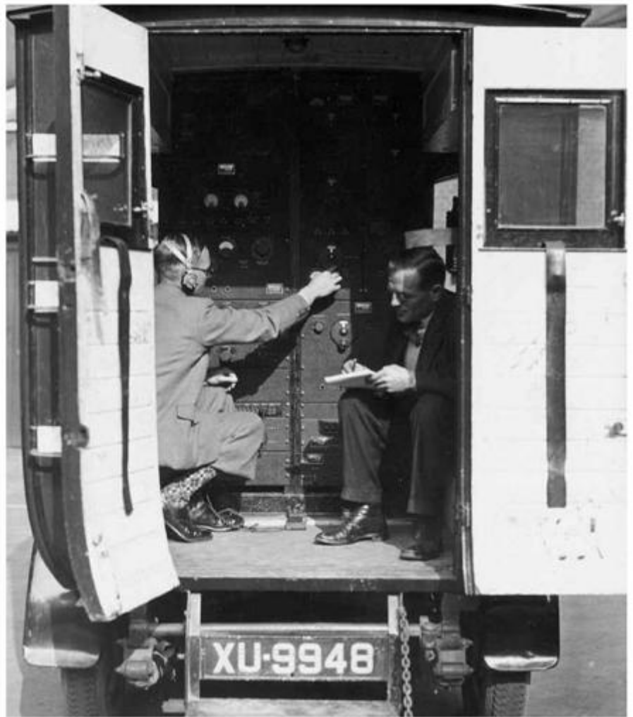
ABOVE: Tuning in – the inside of one of the GPO's wireless detecting vans in the early 1930s.
