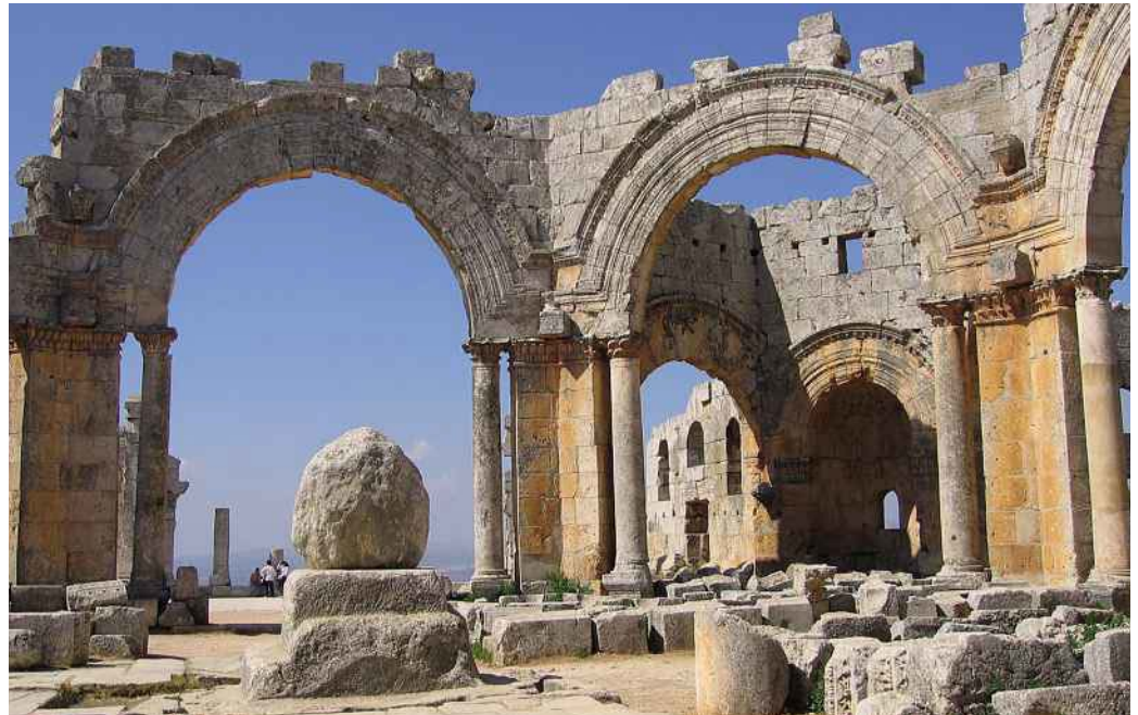
ABOVE: The plinth of Simeon's final pillar, complete with later boulder. BELOW: A recent photo shows severe damage to the plinth.
