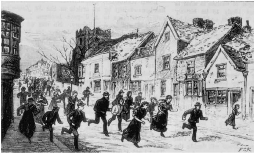
LEFT: Panic on the streets of Colchester during the Essex earthquake of 1884. BELOW: The church at Langenhoe sustained terrible damage.
