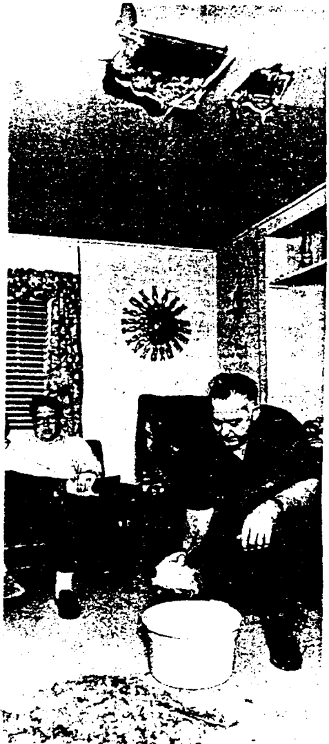
Wilbert Cullers examines part of the ice which came through his roof (Timberville)
