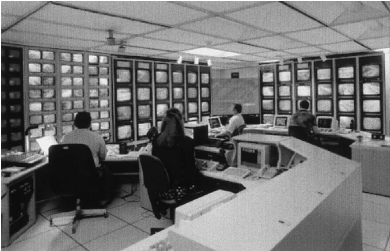
Figure 1. A typical traffic management center. The most visible equipment includes the array of CCTV traffic monitors and the computer consoles for the human operators. (Source: Federal Highway Administration)
