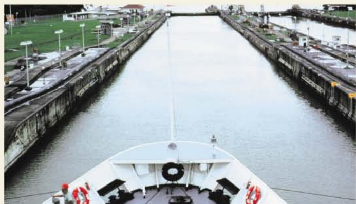
Lock in the Panama Canal, Panama To fit into the canal's locks, ships must be no more than 32.3 m wide and 294.1 m long.
